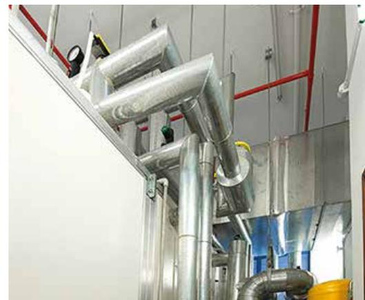
Chilled water ducting with green recycling ability.
